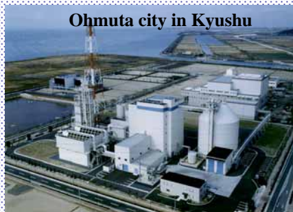
RDF production & combustion - power generation plant
